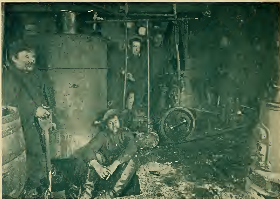
BY JANUARY 23D, OUR LITTLE LIGHTING PLANT WAS COMPLETE AND OUR ENGINEER WAS READY TO ILLUMINATE THE CAMP WITH ELECTRICITY
